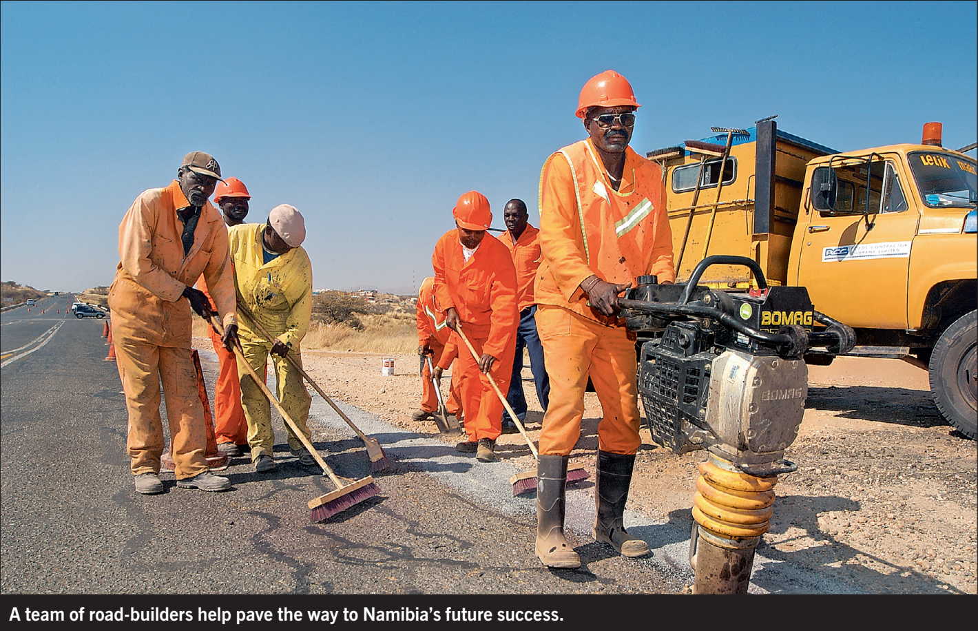
A team of road-builders help pave the way to Namibia's future success.
